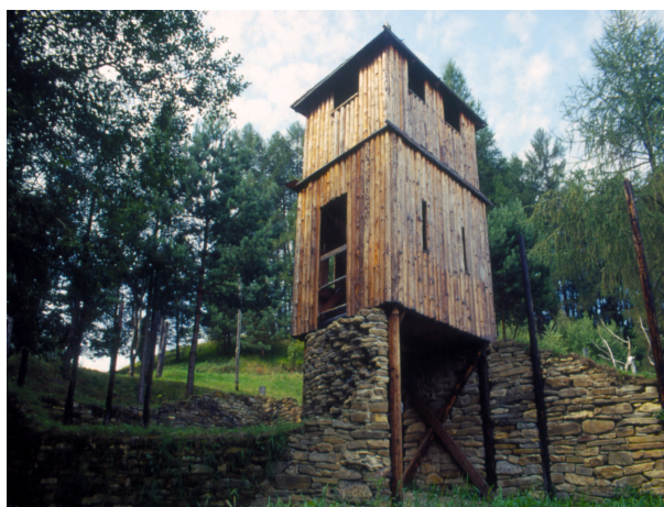
Fig. 4. Finished tower with a partly reconstructed stone masonry wall in its close surroundings in 2007.
