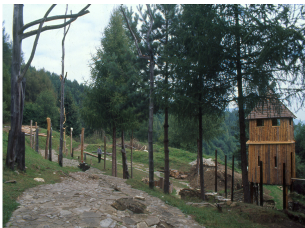
Fig. 6. Finished tower as a part of hypothetically the reconstructed sacred area—insight view from the inner area of the fortress (2007).
