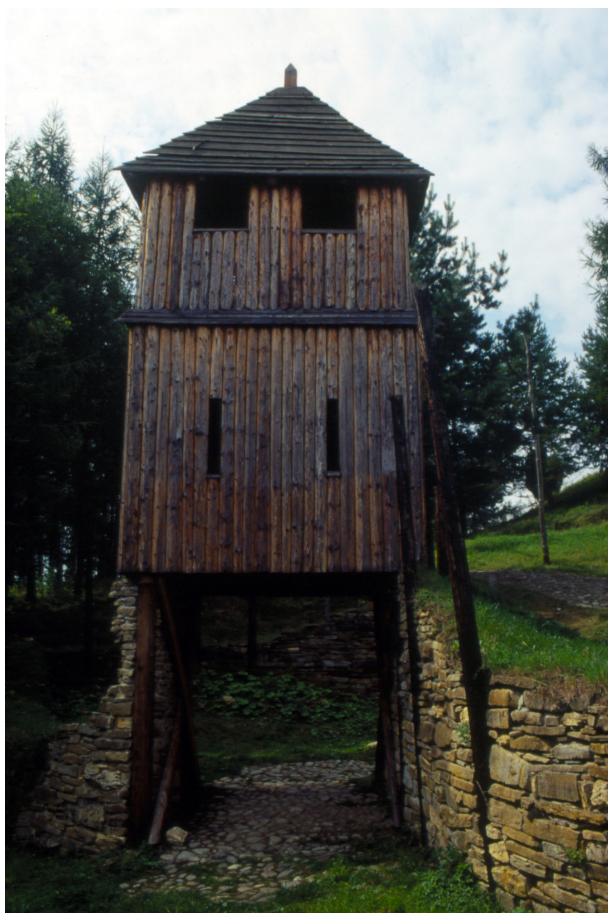
Fig. 5. Finished works on the wooden part of the gate tower to the sacred area – a look through the gate (2007).
